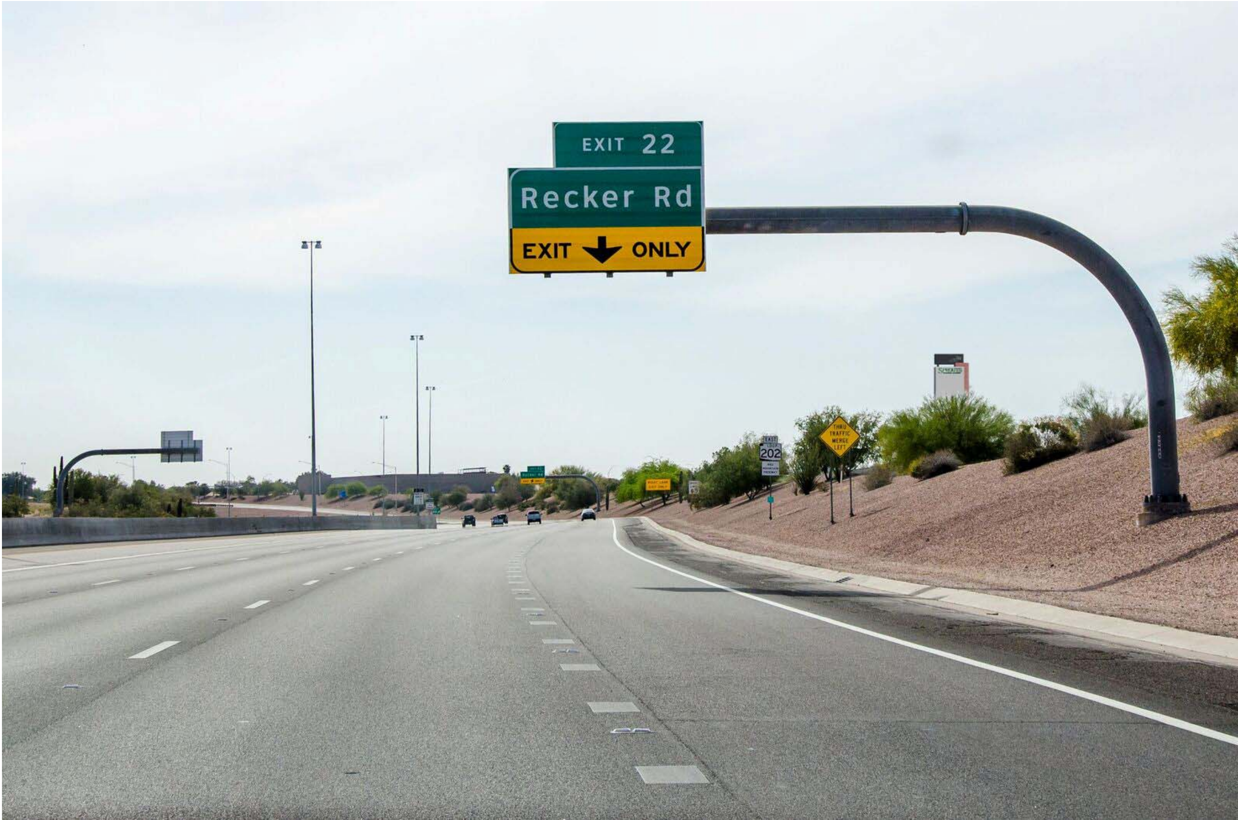
Sign 2: 60ft. Eastbound Just Past Higley On-ramp
