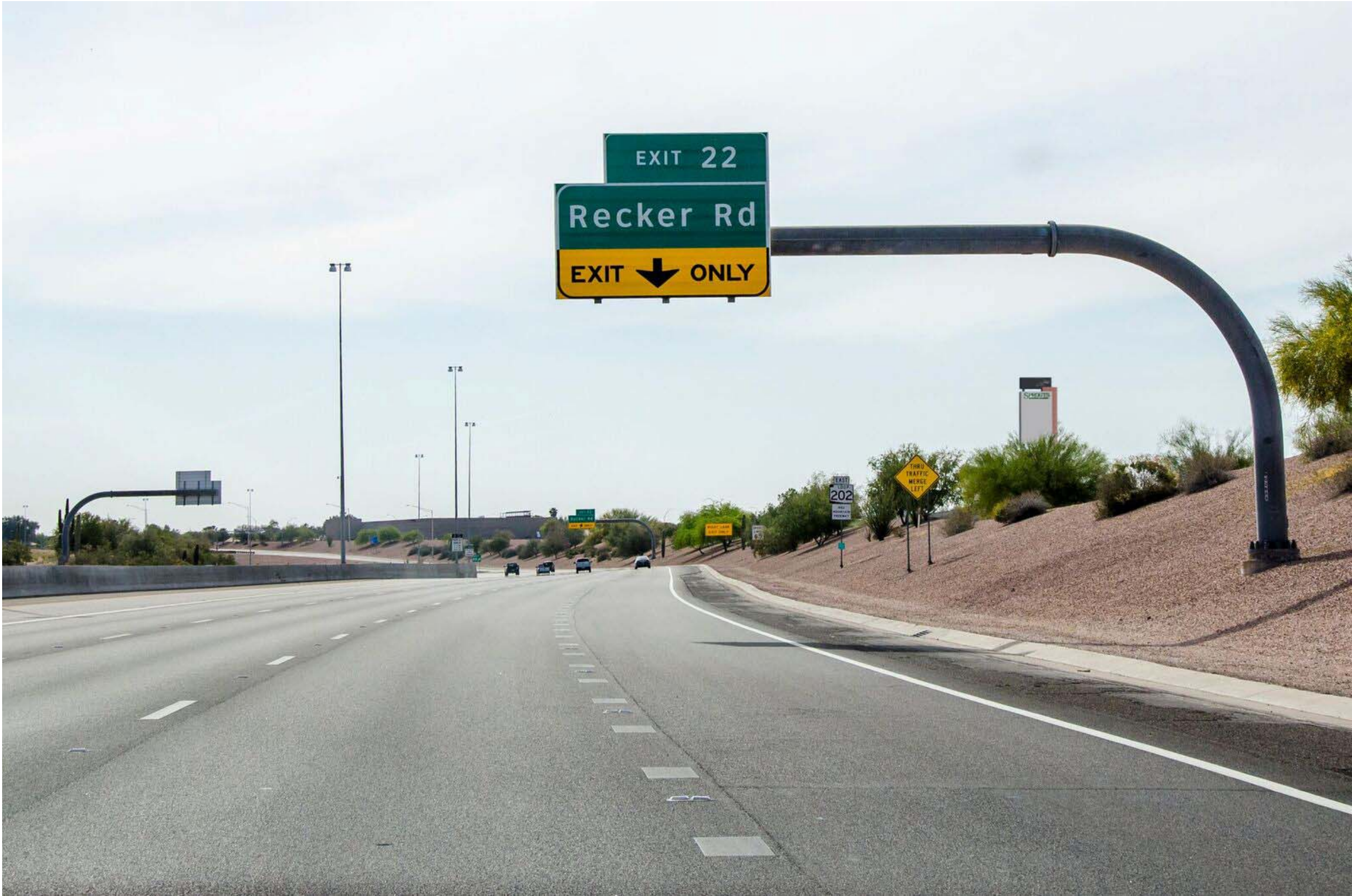
Sign 2: 70ft. Eastbound Just Past Higley On-ramp
